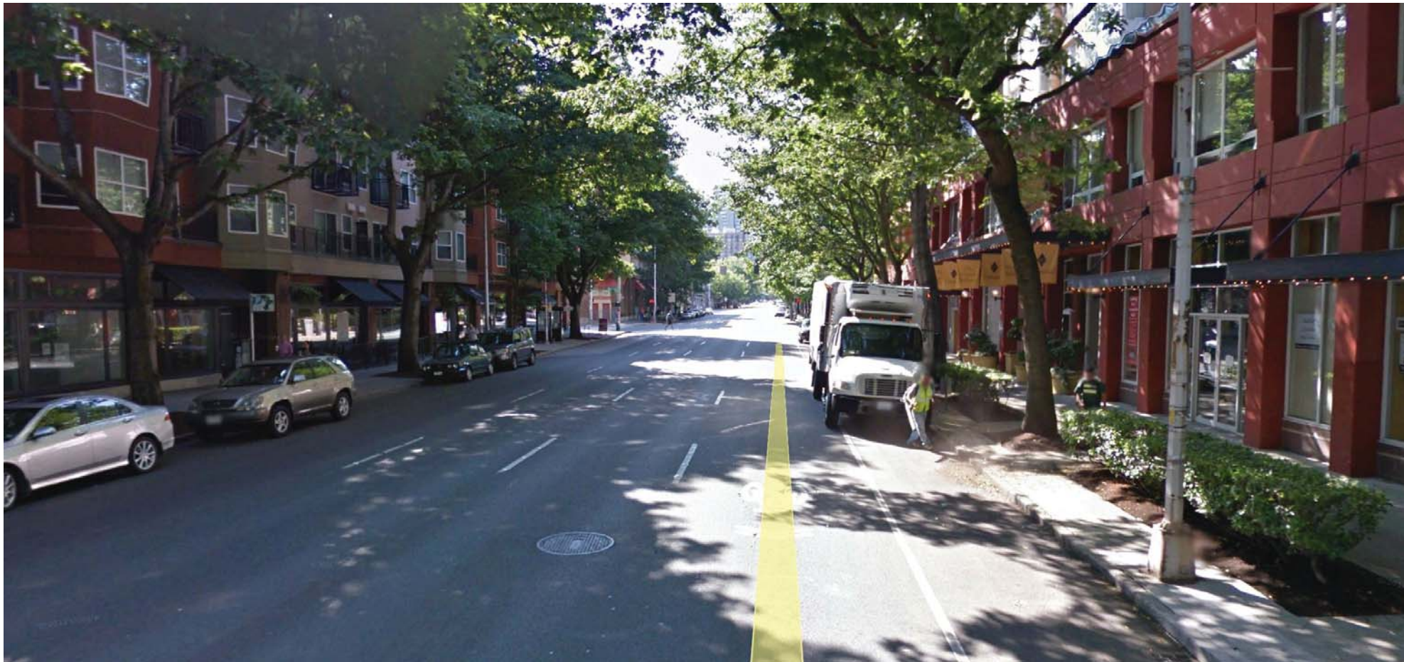
SW Street Perspective View - Centennial Tower Apts (right side of image) The stepped facade allows for healthy canopies to grow on trees, simultaneously allowing the tower to rise high while maintaining a human scale.
